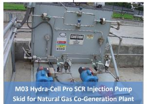
SNCR applications require higher flow rates and pressures, perhaps up to 2000 PSIG. SNCR requires injecting urea or ammonia into the flue gas at high temperature 1600-2100°F). (typically atomization and even distribution are critical since there is no catalyst to promote the reaction. These droplets need to evaporate uniformaly within а residence time. This differs from SCR where the reagent is applied to the surface of the catalyst and atomization is less critical.
